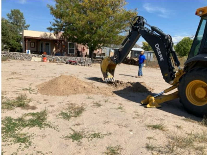
The open space to the south of Stephanie McReynolds' house. San Ildefonso Pueblo's facilities department staff are testing the soil at the proposed location of the new drain field.
