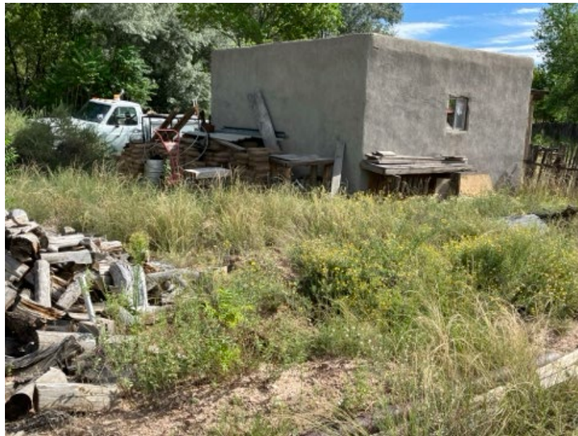
The existing septic tank located near this shed will be crushed and abandoned in place.
