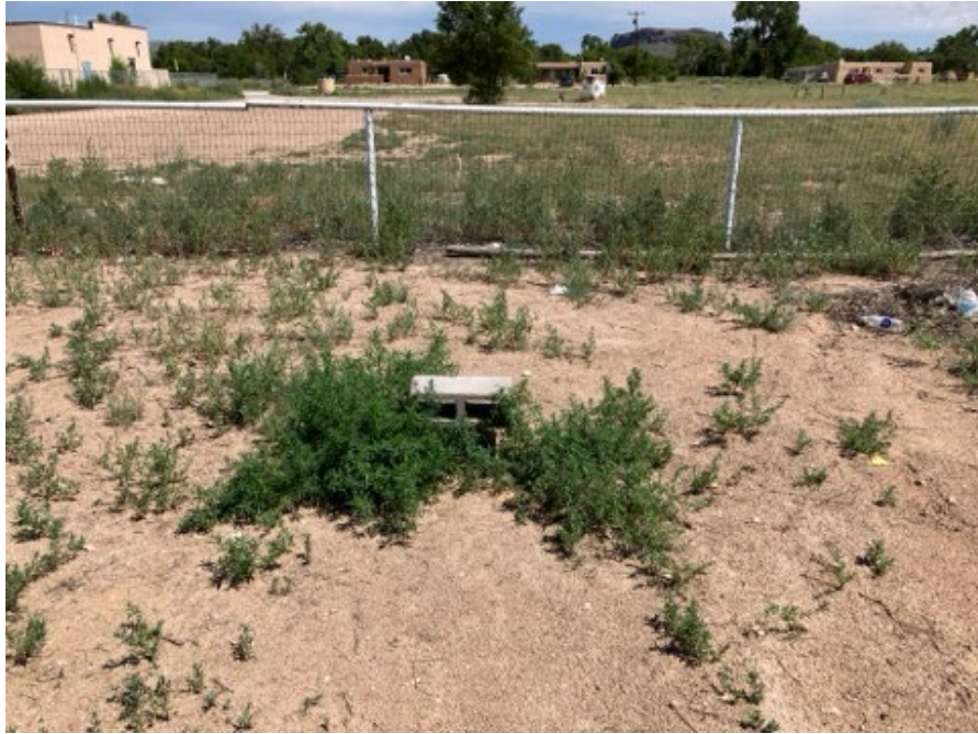
An existing SSL cleanout located north of the house. The existing SSL line will be capped and abandoned in place at this location.
