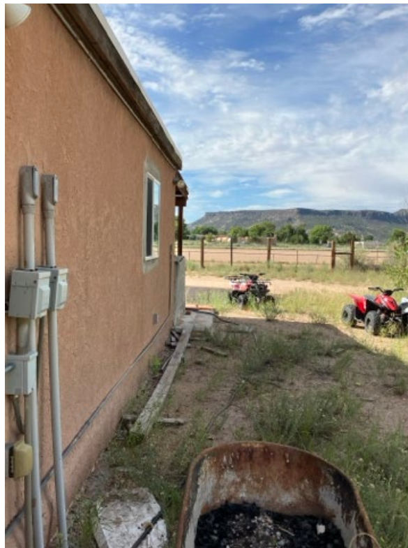
View of the west side of the house. The new effluent line will run parallel to the house, offset about 10 feet.
