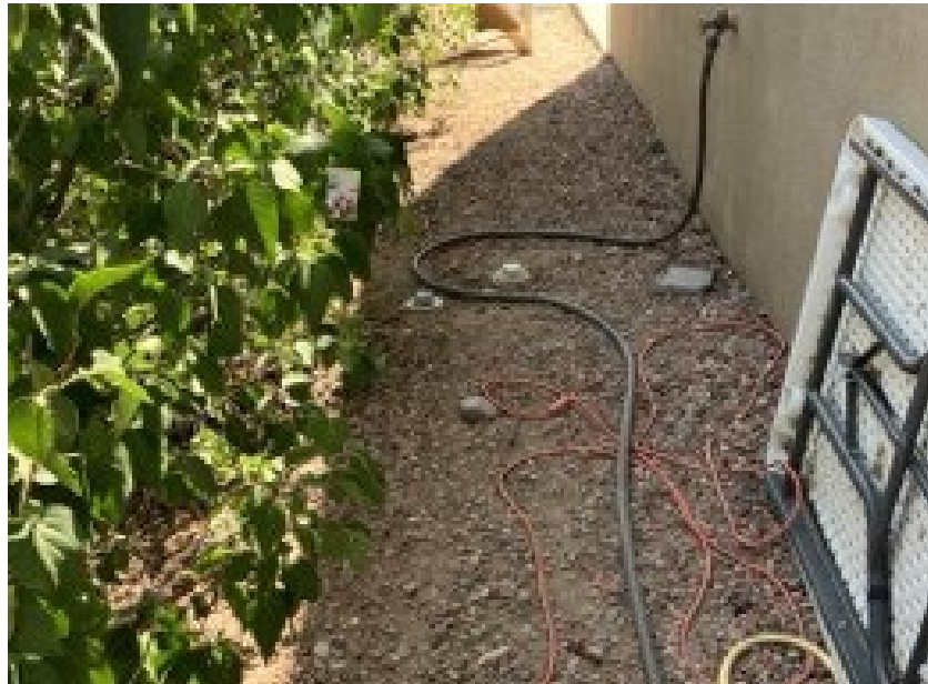
View of the existing sewer service line (SSL) cleanout at the north wall of the house. The new SSL will connect to the house at the same location.
